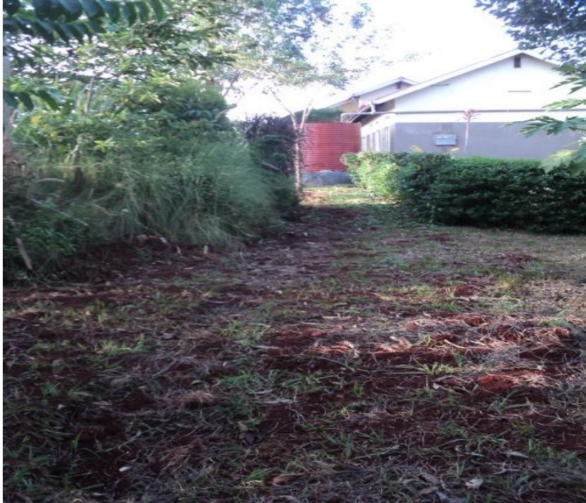
Figure 5: Fresh soils show half the distance from the tap in the compound to the building. With the JWF, the water was extended up to the building
