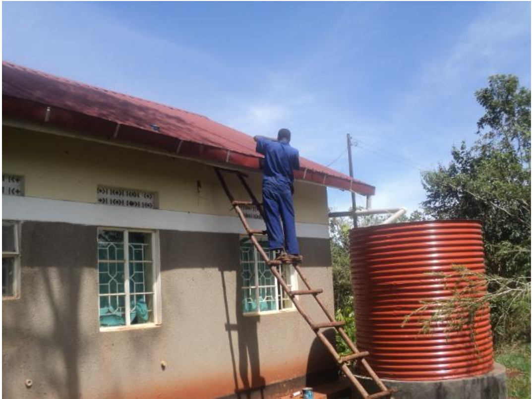
Figure 2: Mr. Muzaale fixing the gutters
