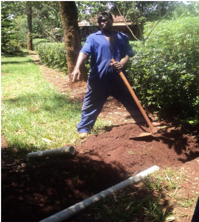
Figure 4: Digging the trench to protect overflowing water away from the building
